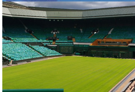
The actuation systems that close the Wimbledon roof and get planes off the ground
