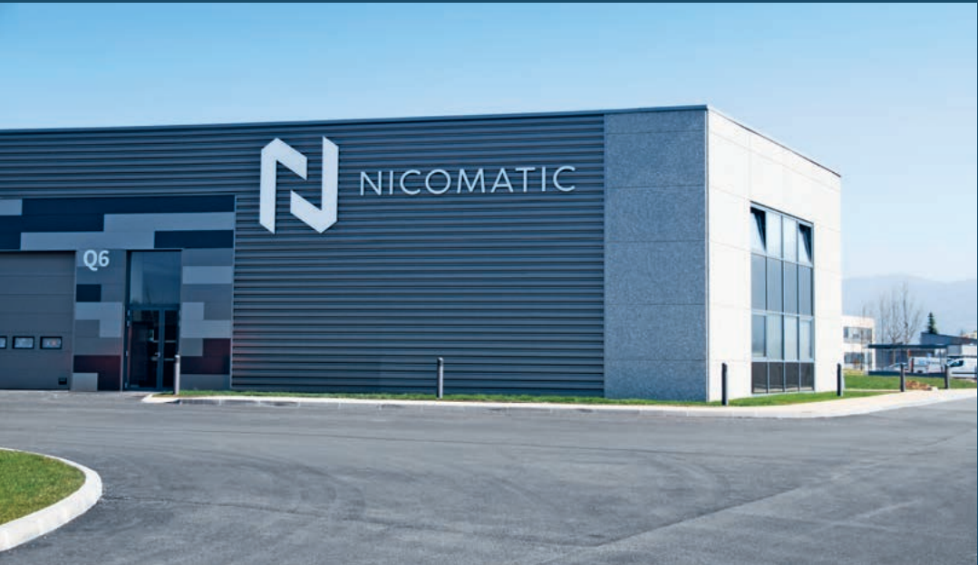
Nicomatic SA’s headquarters in Bons-en-Chablais is one of several production sites where connection solutions are manufactured for customers worldwide.
